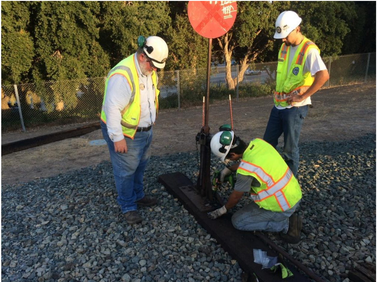
Frank, Josh, and Matt make the final adjustment to the head-block at Switch 16
