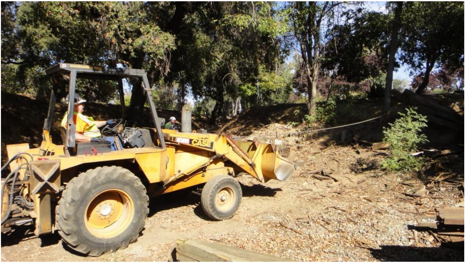
Harry and Frank use a chain to pull a buried bridge timber from the pile
