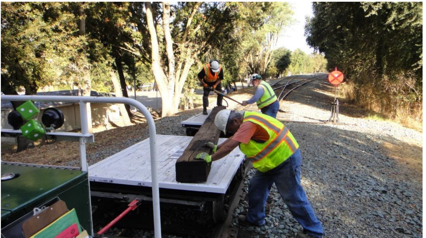
John, Fred, and Frank load the old head-block from Switch 16 on the flatcars
