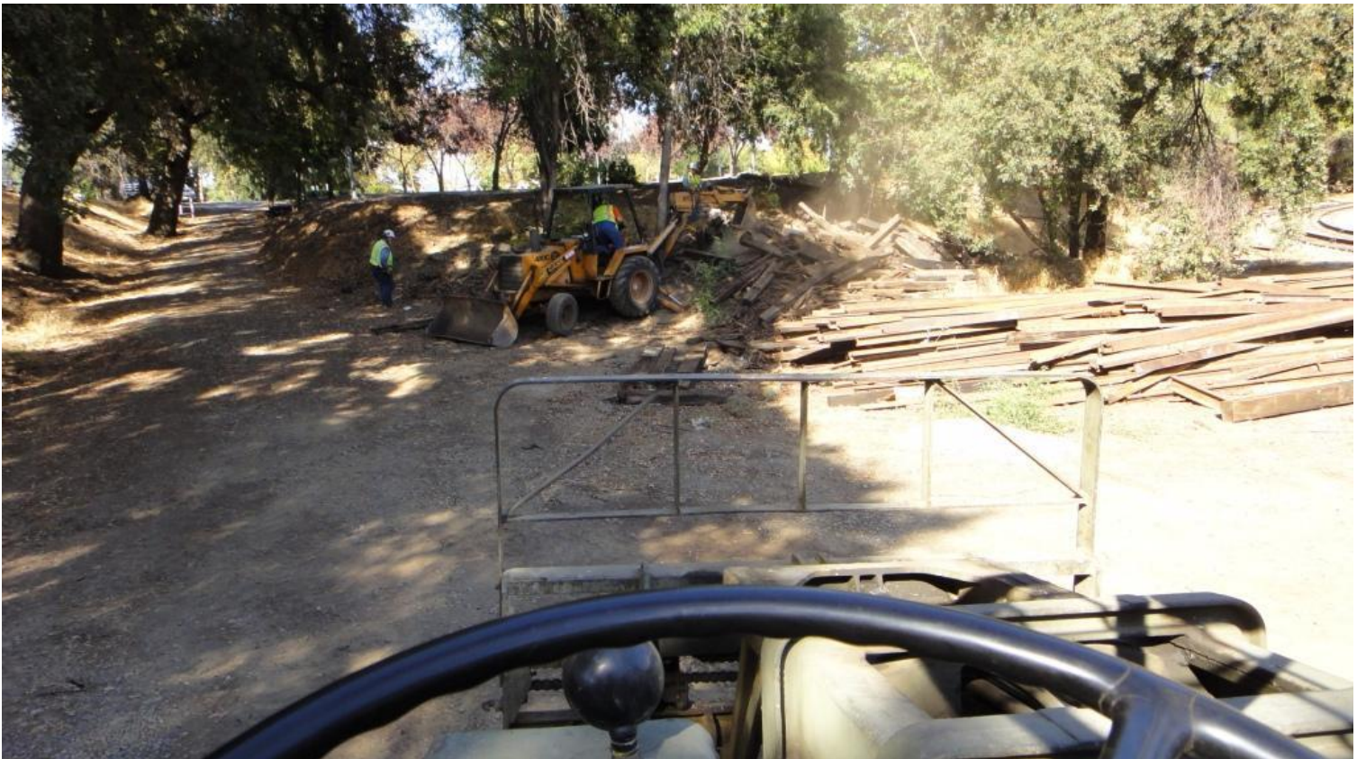
Our expert back-hoe operator, Harry, uses the "Extendahoe" to pull the pile into position for the Big Green Machine to grab the ties
